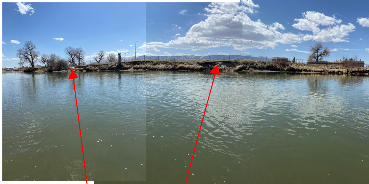
Photo 1: View south looking across the river at the unstable river bank adjacent to the Sam H. Hobbs Regional Wastewater Facility
